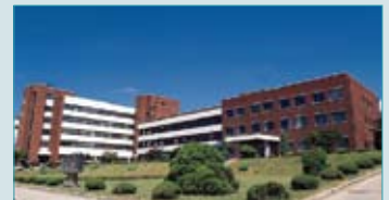
Former Research Center
