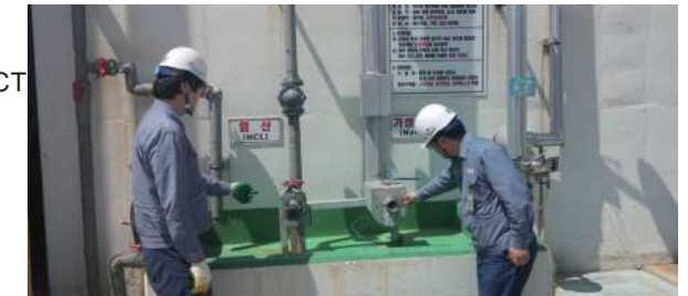
Checking hazardous chemical substance facilities
